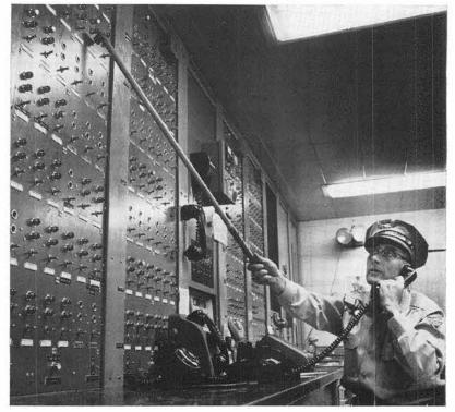
INTRUSIONS of alarmed buildings, repositories, and other sensitive areas during non-working hours are indicated immediately on this panel in Bldg. 801. Danny Stringfellow (3242) takes a call from a security inspector while switching off a panel light.
